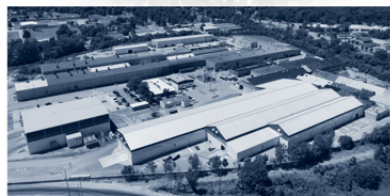
Fort Wayne plant, IN-USA
